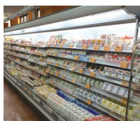
CO 2 refrigerant based refrigerated open showcases
